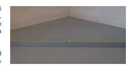
Pay attention to the specific properties of each screed (Installation maturity is achieved when the moisture content measurement yields values of 1.8 % for cement and 0.3 % for anhydrite screed, ...). Existing features of the sub-floor, such as construction / building gaps or expansion gaps in the screed, should not be altered when laying your new floor.
